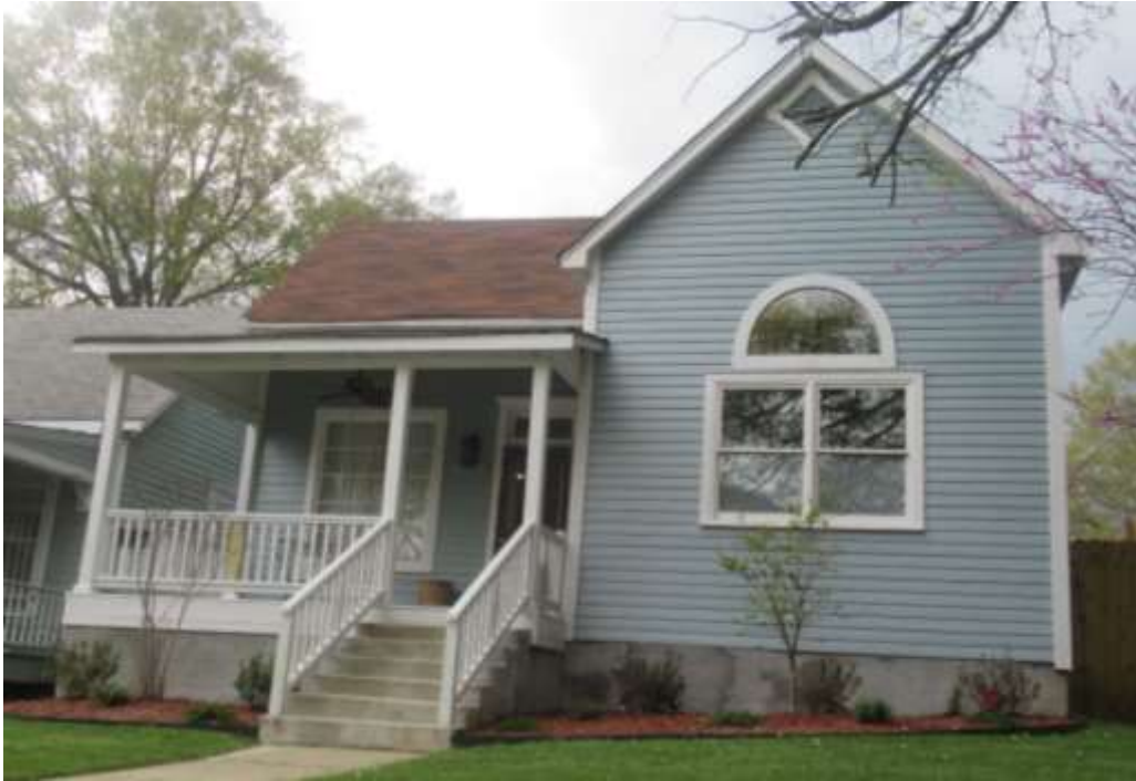
March 2018 – work complete
