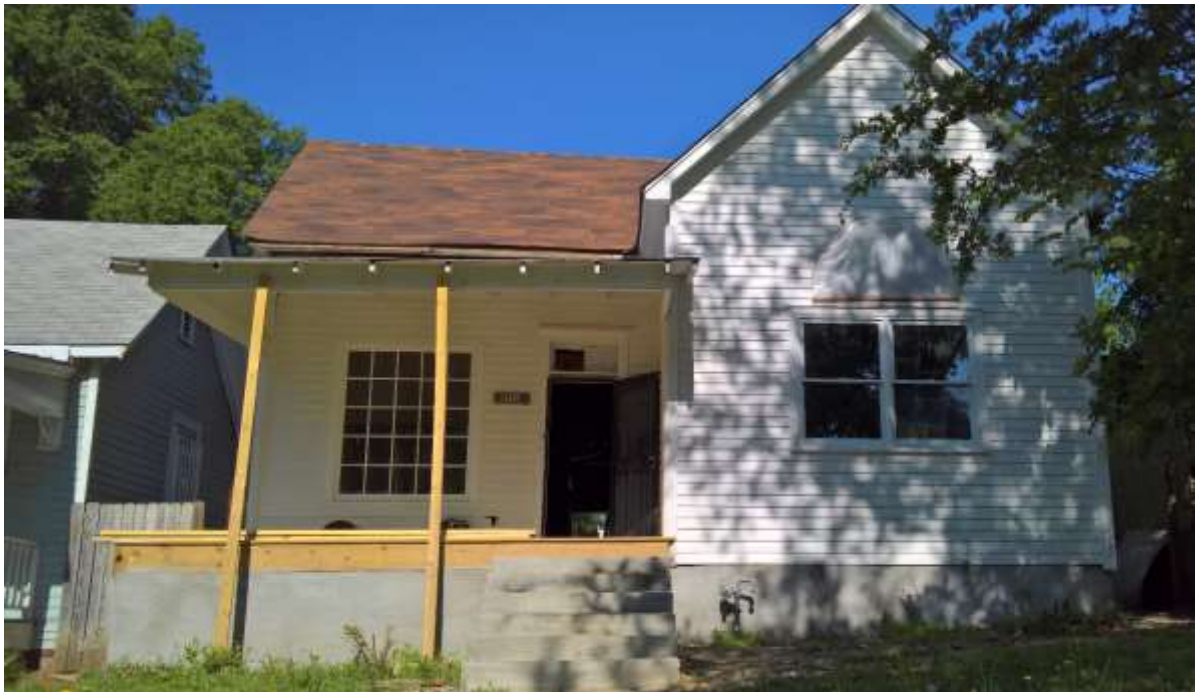
April 2017 – work in progress
