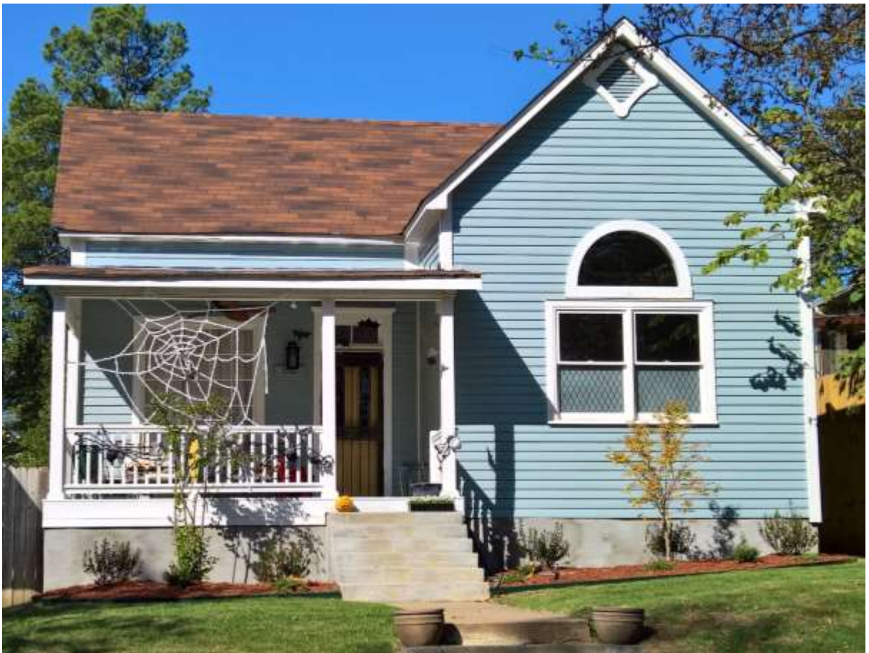
October 2017 – work complete
