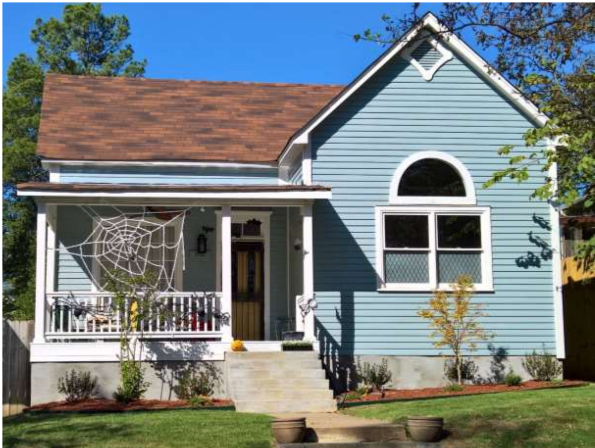
October 2017 – work complete
