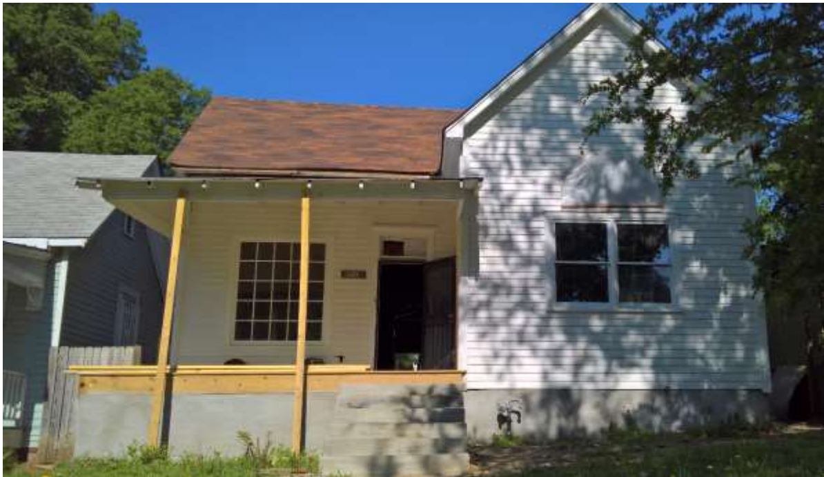
April 2017 – work in progress
